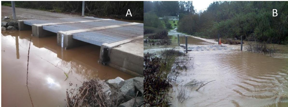
Figure 11: A) New box culvert beneath Sill Road. The white rectangle in the center of the picture is a staff plate. Black cylinder on the right side of the image is the stilling well for the pressure transducer of the Sill Road gage (Fig. 8). B) Same view as Figure 9 during 12/12/15 flow of 2014. Flow rate is approximately 90 cfs, corresponding to an exceedance recurrence interval of less than 0.5 years.
