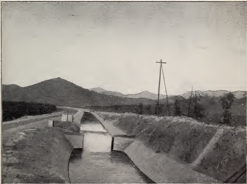
FIG. 2.—DIVISION BULKHEAD OF GAGE CANAL, CALIFORNIA.
