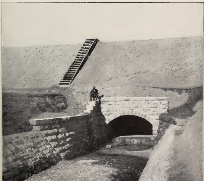
FIG. 2.—OUTLET CONDUIT NO. 2, GREAT PLAINS WATER COMPANY.
