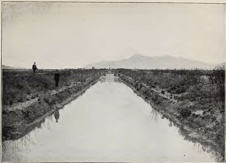
FIG. 1.—BEAR RIVER CANAL, LOOKING NORTH, SHOWING DROP.
