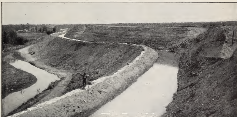
FIG. 2.—SIDE HILL CONSTRUCTION ON AN IDAHO CANAL.
