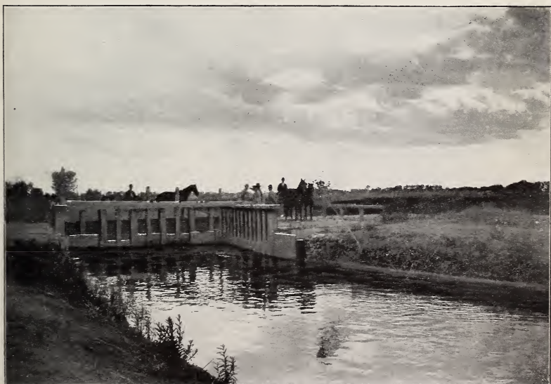
FIG. 2.—DIVISION GATE OF THE CONSOLIDATED CANAL COMPANY, ARIZONA.
