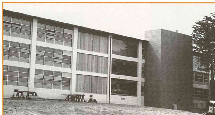
Building 47, home of the new Campus Service Center.
