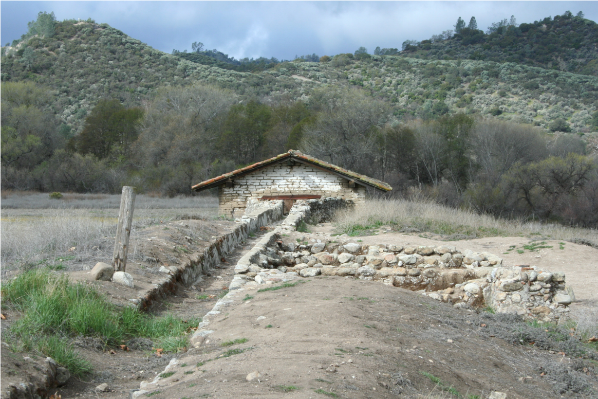
Irrigation system leading to the tannery and 1806 grist mill. Facing west. March 14, 2012.
