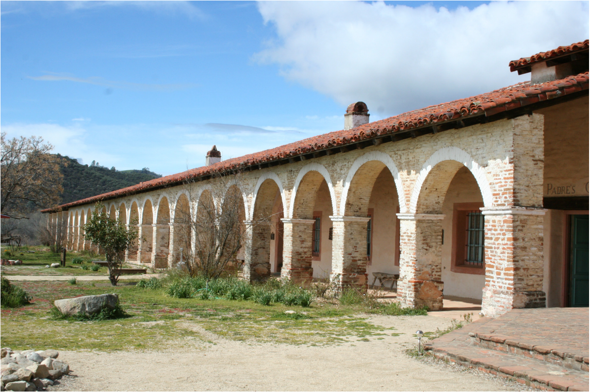
View of the front elevation arcade. Facing west. March 15, 2012.
