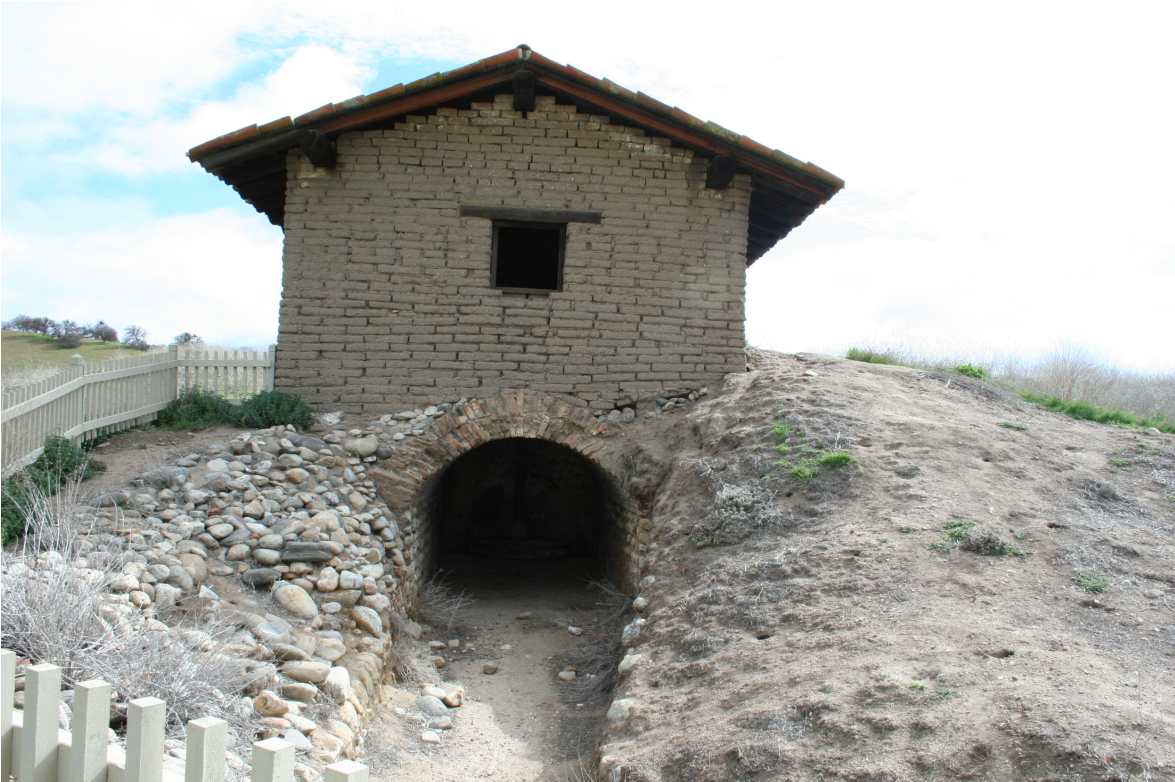
Restored 1806 grist mill. Facing east. March 14, 2012.
