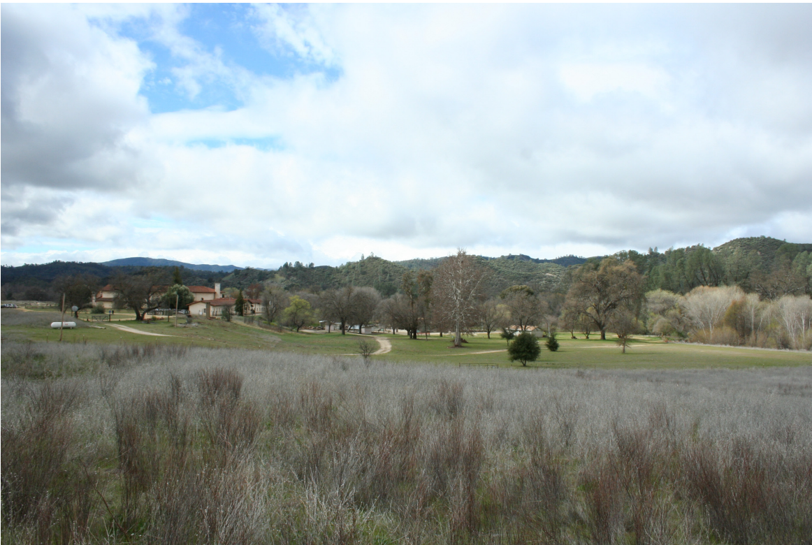
View of the east (side) elevation from Mission Road. Facing southwest. March 14, 2012.
