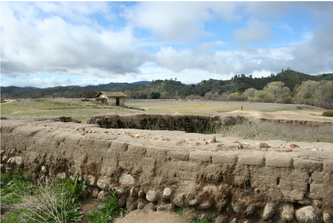
Wall of the Indian Cemetery, laid out in 1804. Facing southwest. March 14, 2012.
