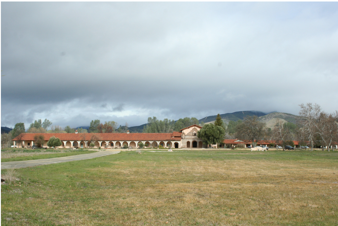
View of the façade of the Mission. Facing northwest. March 14, 2012.
