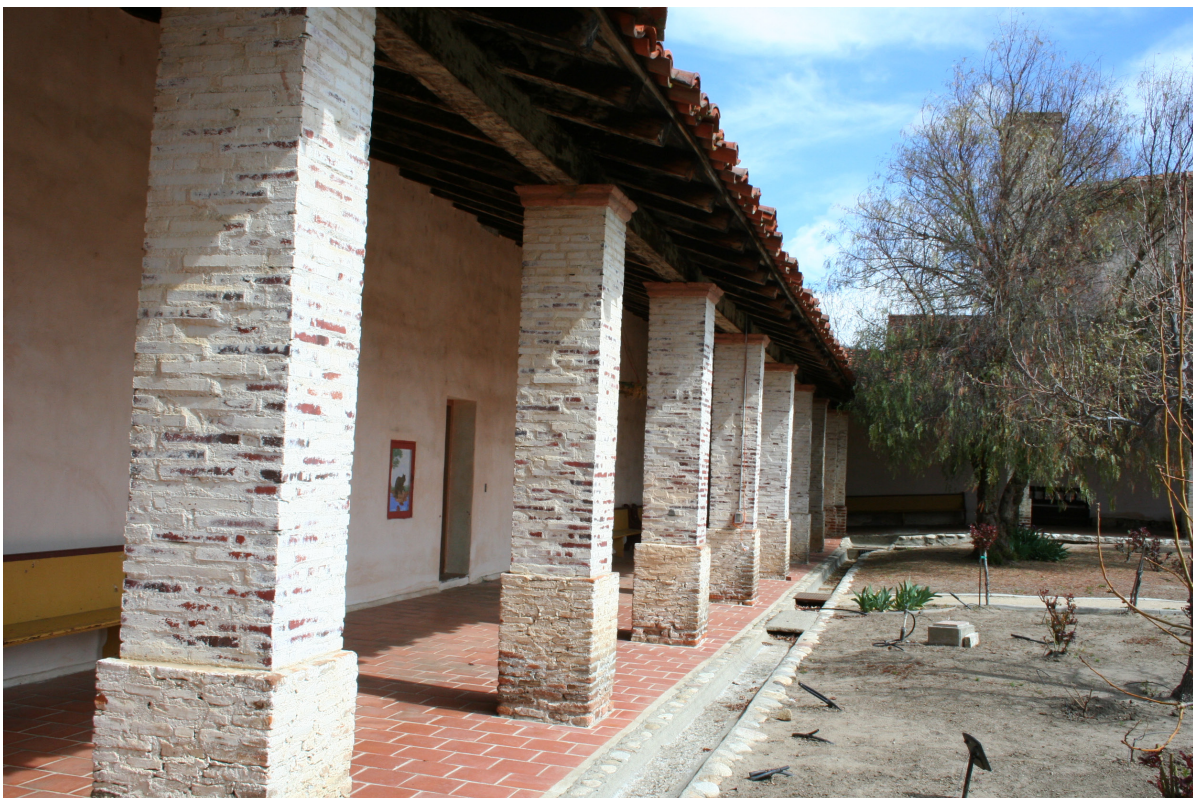
Brick columns and arcade in courtyard and courtyard water feature. March 15, 2012.
