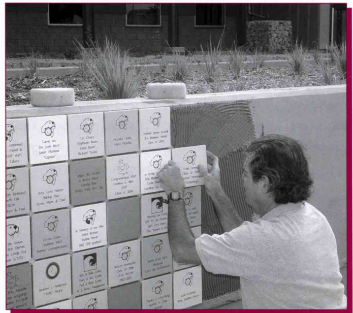
Installing the first tiles on the courtyard wall
