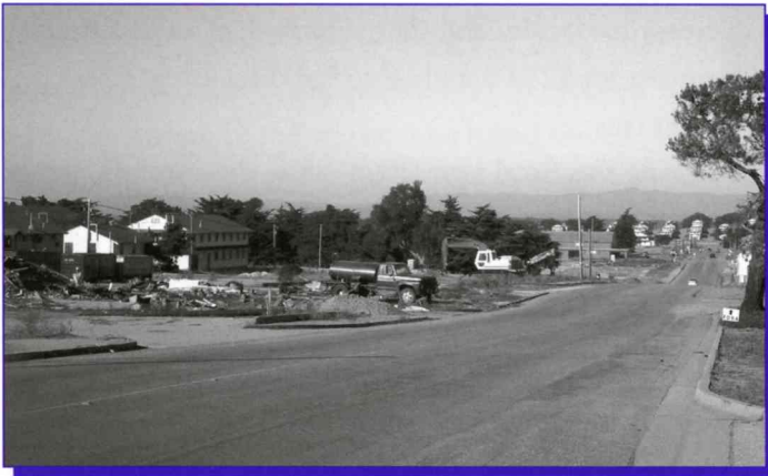
Site of demolished buildings along Second Avenue, looking north
