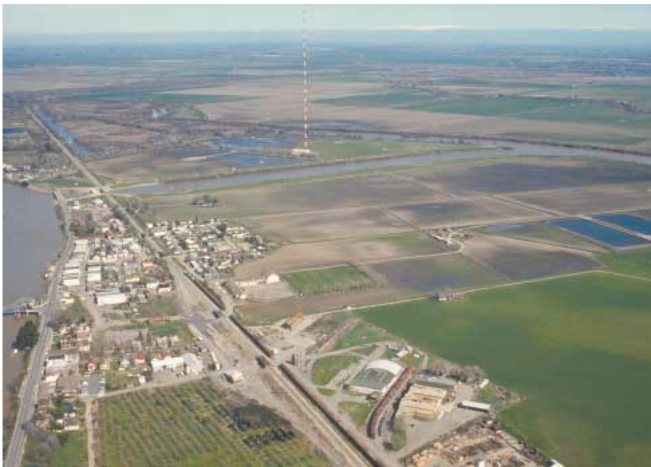
The Delta Cross Channel, a CVP facility constructed in 1951, was designed to help move water from the Sacramento River into the southern Delta. A gated inlet structure (left side of photo) on the Sacramento River about 1 mile north of Walnut Grove is operated to divert river water into a 4,200 foot-long channel connecting the Sacramento River to Snodgrass Slough, part of the Mokelumne River system. Maximum diversion capacity is about 3,500 cfs. SWRCB Order WR 95-6 requires that the Cross Channel gates be closed more frequently, to keep migrating salmon in the Sacramento River.
