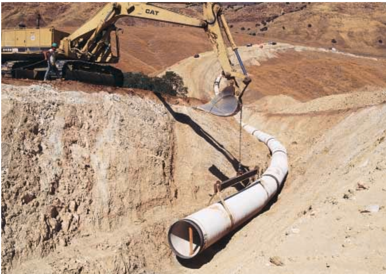
Completion of the remaining 100 miles of the SWP's Coastal Aqueduct from Devils Den to the Santa Maria area in Santa Barbara County links the southern half of the central coast region to California's system of major water infrastructure.
