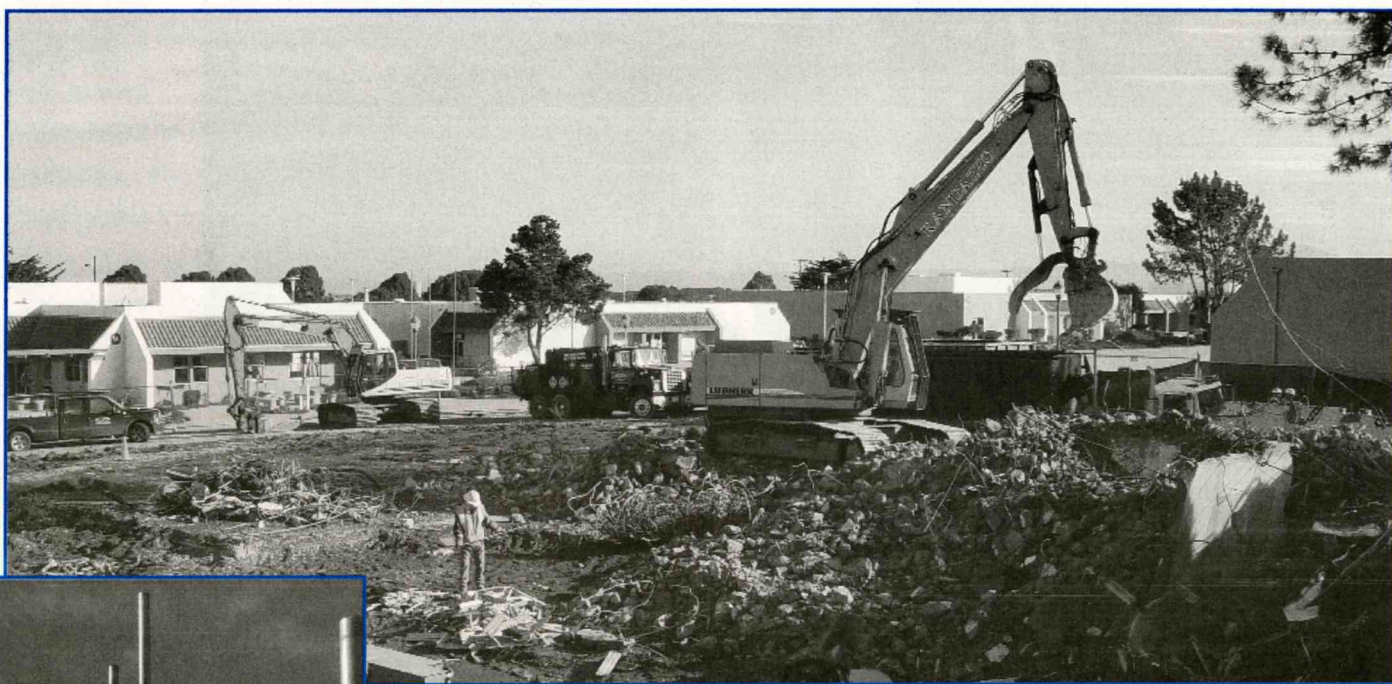
The remains of Bldg. 207 as it's demolished during the winter break.
