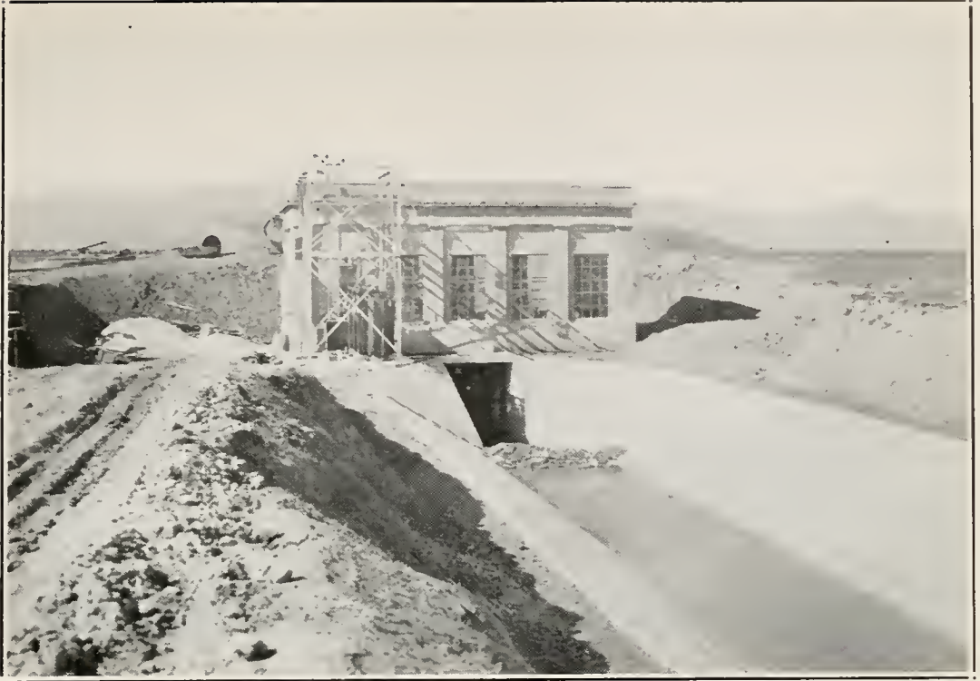
FIG. 1. A principal pumping plant in West Stanislaus Irrigation District.
