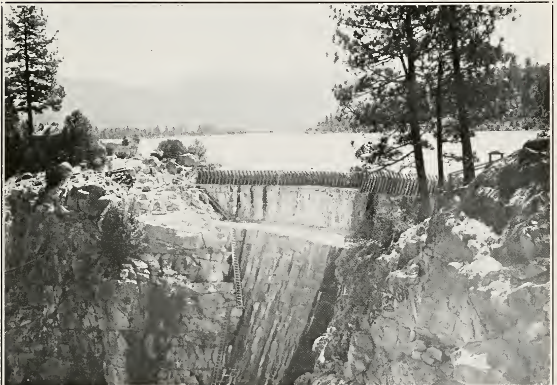
FIG. 2. Hemet Dam and Reservoir, principal source of water for lands in recently organized Hemet Irrigation District.
