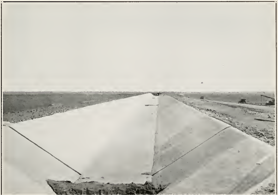
FIG. 2. Concrete-lined main canal, West Stanislaus Irrigation District.
