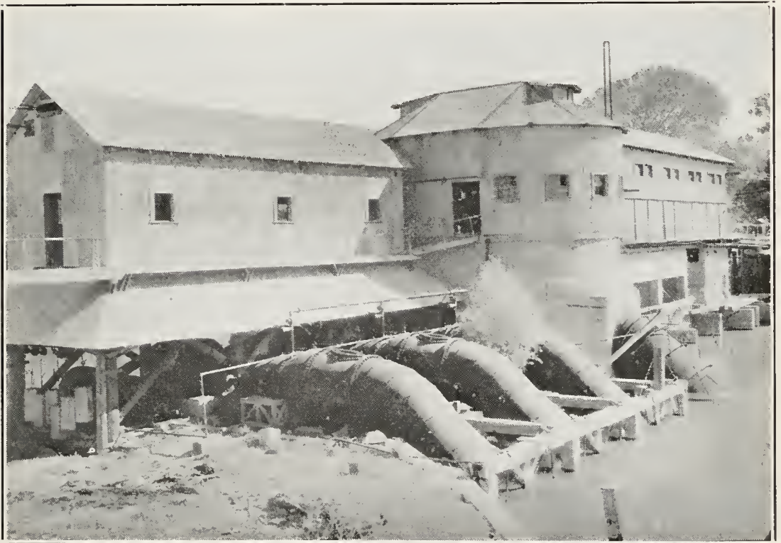
FIG. 2. Pumping plant of Glenn-Colusa Irrigation District for diverting water from Sacramento River into Central Canal.
