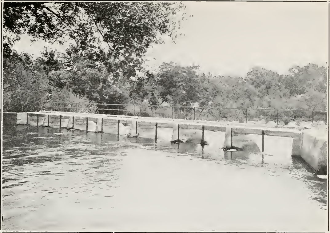
FIG. 1. Weir across Kings River at head of Gould Canal, Fresno Irrigation District.
