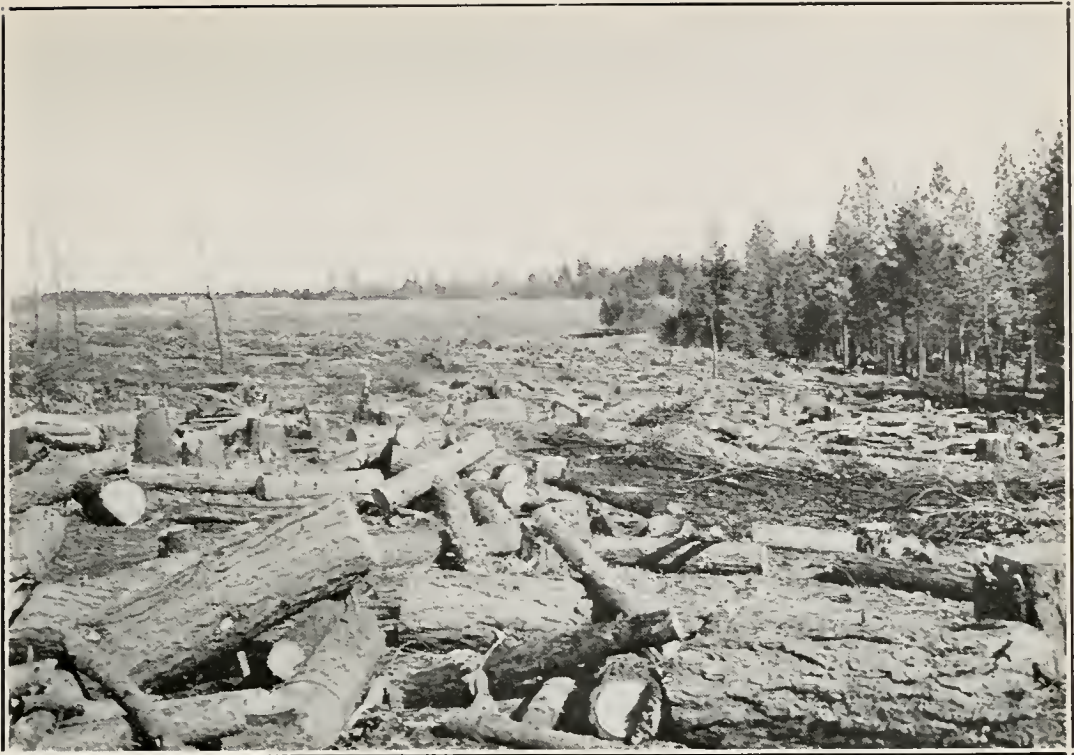
FIG. 1. Clearing land in typical portion of the upper area of Nevada Irrigation District.
