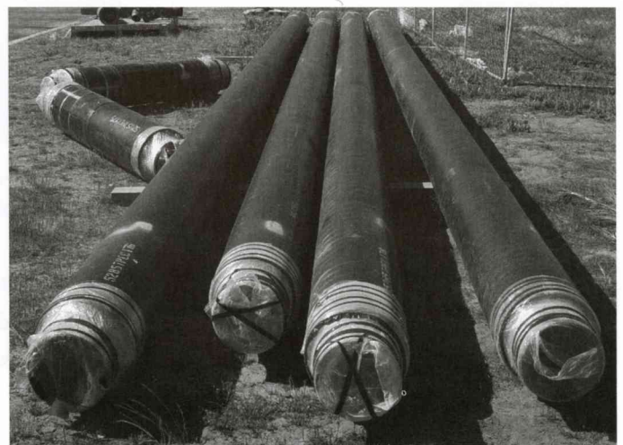
Ranging from six to 16 inches in diameter, the steel hot water pipes are heavily insulated to minimize heat loss.
