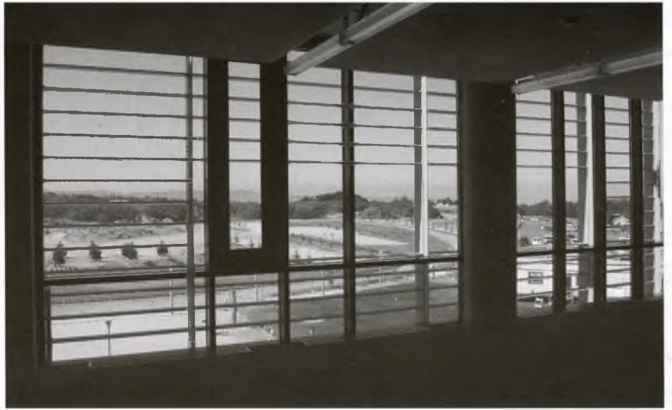
View from the Archived Reading Room on the third floor overlooking the crescent. Horizontal louvers allow sunlight to enter but shade the interior to reduce the need for air conditioning to save energy.
