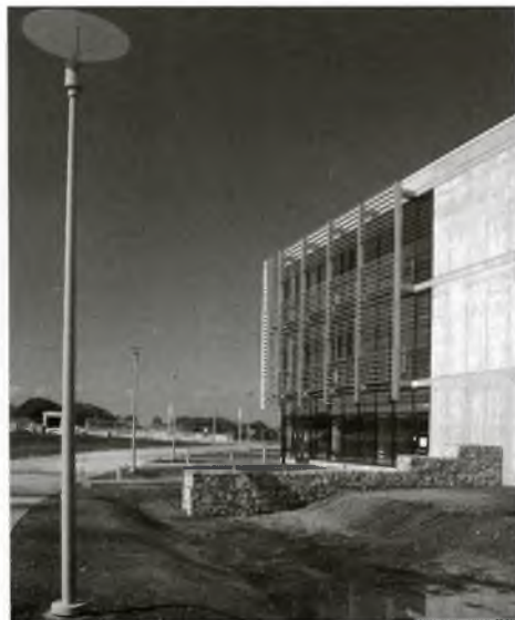
A rock wall dissipates the energy of water collected from the roof, discharging it into a pond where it percolates into the soil to replenish the aquifer. No runoff enters campus storm drains.
