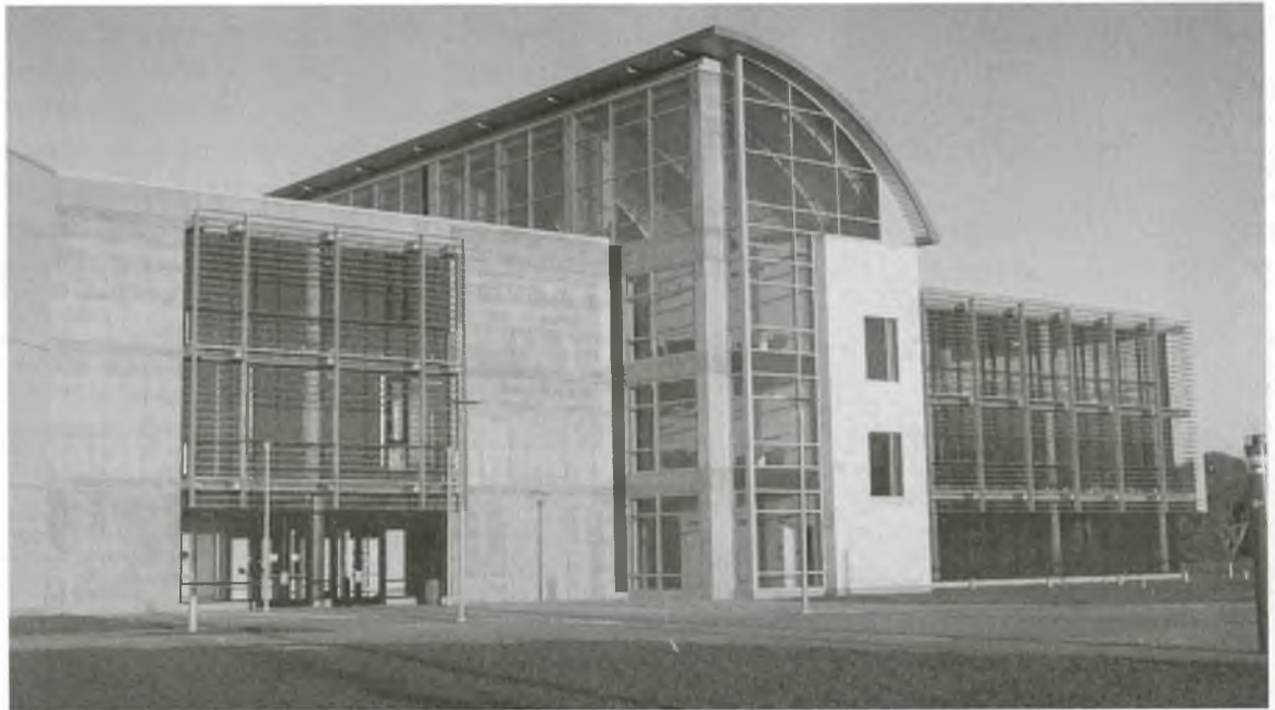
View of the southwest side of the library, facing the crescent, with its large patio area in the foreground.
