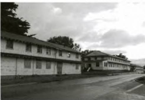
Divarty Street at Second Avenue before demolition work began.
