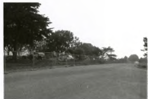
At press time, the demolition work and removal of debris was almost completed.
