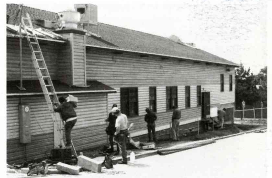
Extensive renovation of the BBC took place during the summer of 2001.
