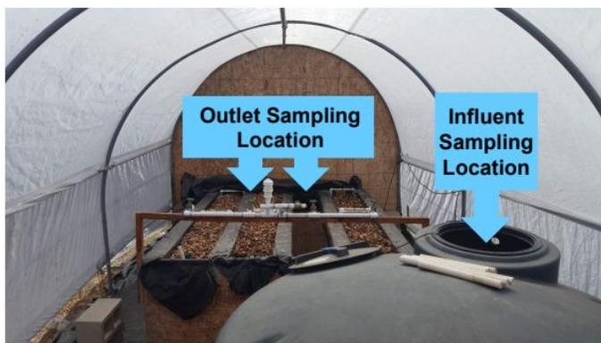
**Figure 1.** The inside of a bioreactor. Note the hoop house structure which helps maintain heat.
